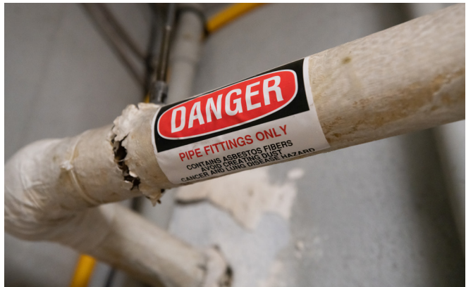
The buildings have the original steam radiator heating systems, the temperature of which cannot be controlled, turning some classrooms into virtual saunas. There are no cooling systems. Roof and skylights leak.
